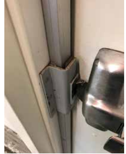
Figure 2: Proper installation of security bracket
